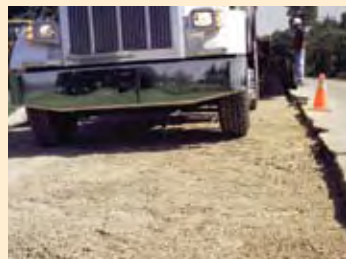
One hour after pouring, 4F Base is strong enough to support a 32-ton vehicle.
